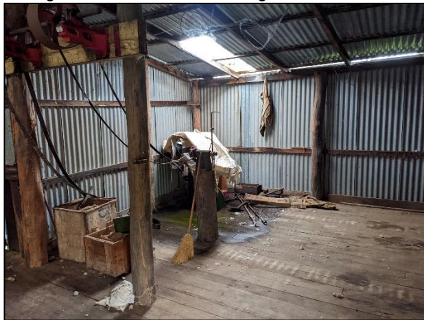
Internal area of western shearing shed
