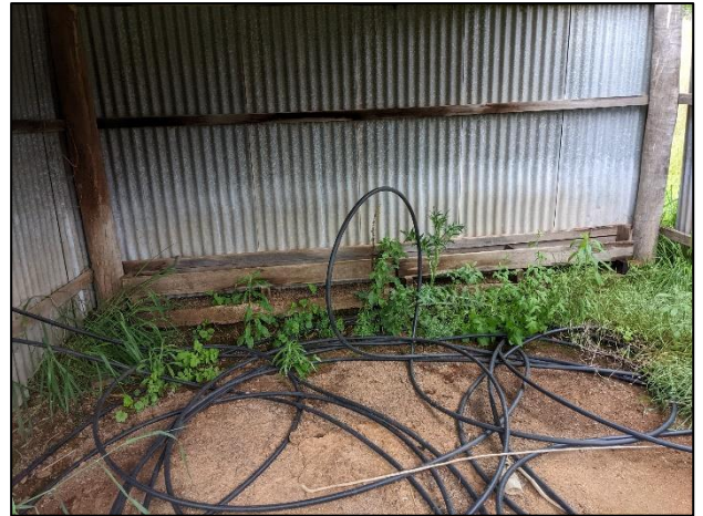
Internal area of southern animal shelter
