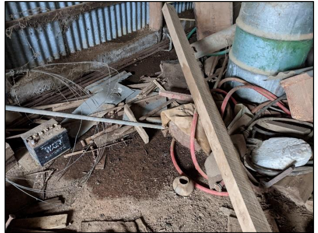
Stained area in western shearing shed
